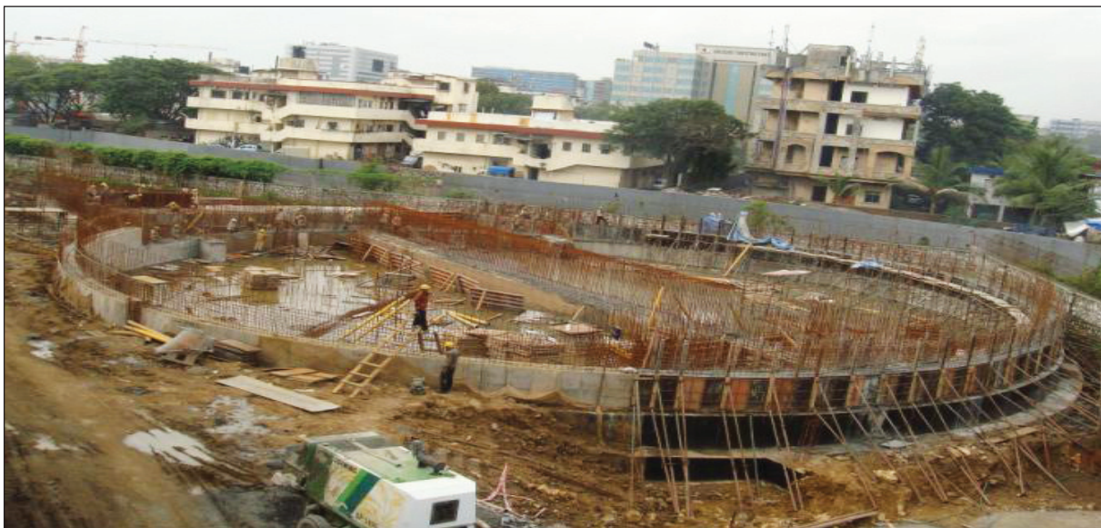
Figure 9: CASS™ Plant under Construction at Mumbai International Airport, Mumbai
